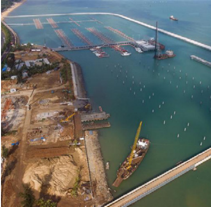
Photo above: Haikou Marina under construction in Hainan Province.
